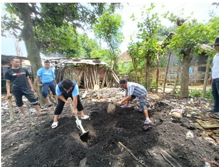
Figure 8. Construction of a Communal Disposal Site (Bruk-Brukan) in RT 003 as a form of Infrastructure Independence
